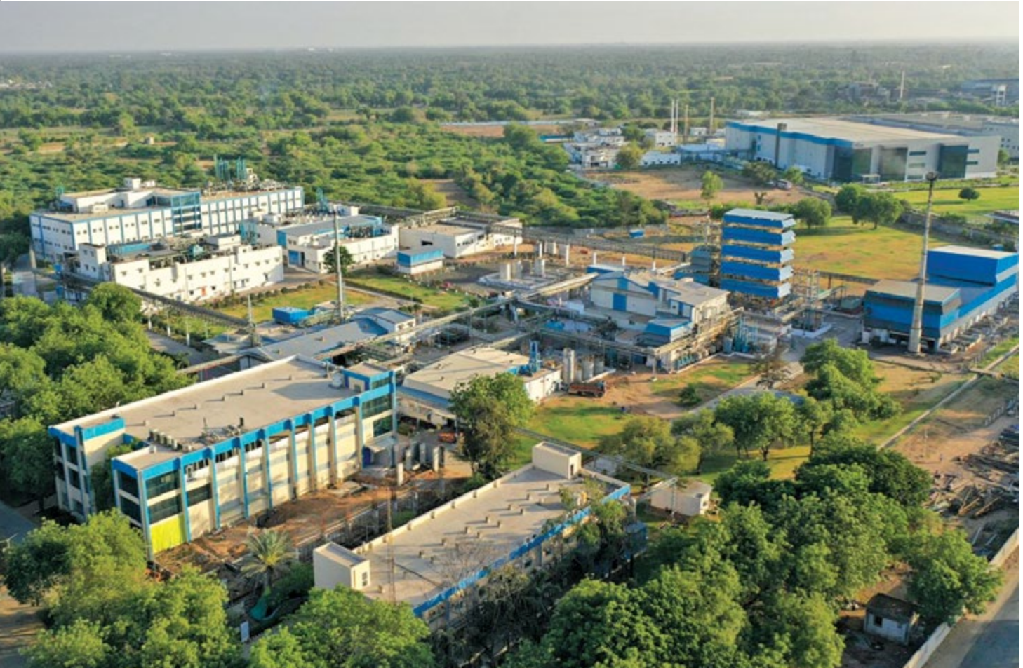
API plant, Karkhadi
